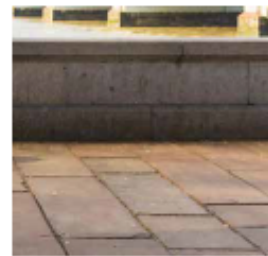
Stone Cladding Sea Wall Development Side
